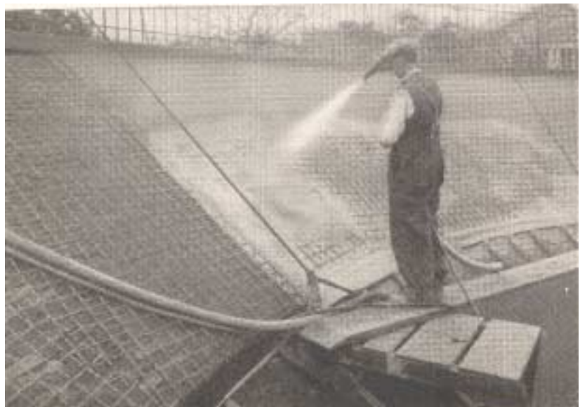
Figure 2. Nozzlemaster applying "Guniting" for a water storage facility in Pittsburgh, 1919.
